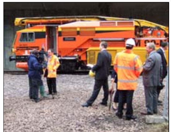
Olwen the Ballast Cleaner at the Start of Works
