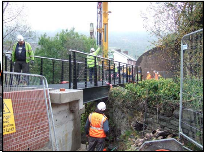
Footbridge being installed at Ebbw Vale Parkway
